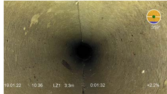
Fig. 6: Example of clean channel (after cleaning)
