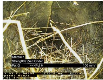
Fig. 10: Example of hair roots growing into the channel
