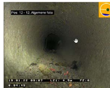
Fig. 7: Example of typical sediment layer < 2cm
