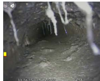
Fig. 8: Example of sediment layer > 2cm
